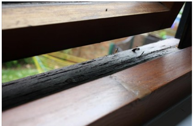
External & Internal 1st floor window
