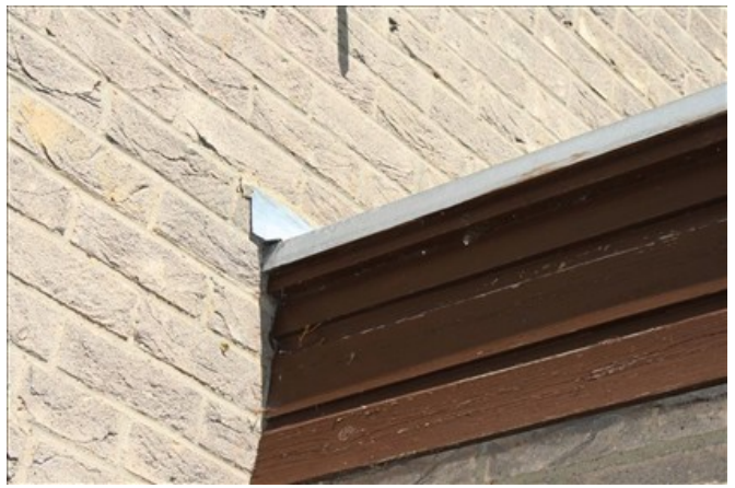
Timber board to edge of flat roof
