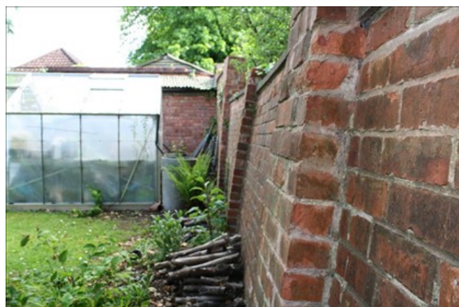
Rear boundary wall
