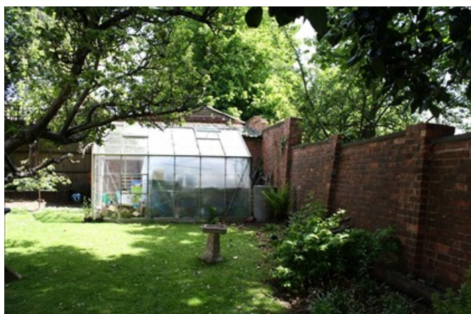
Rear boundary wall
