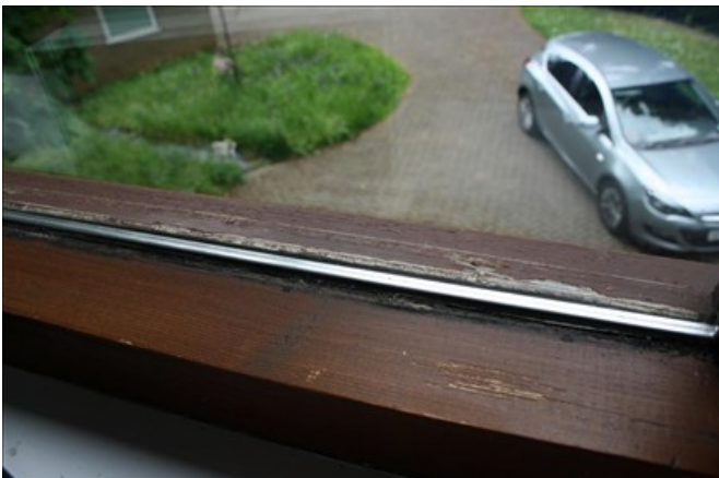
Internal 1st floor window
