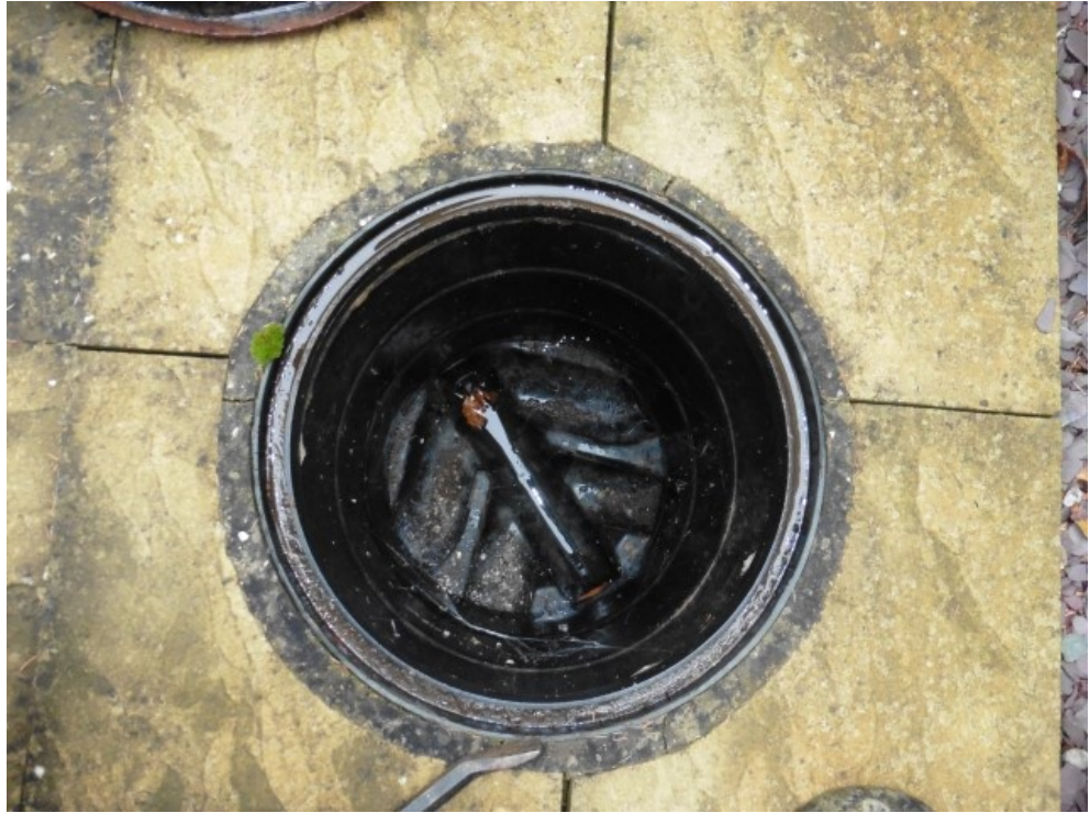
Inspection chamber to the front
