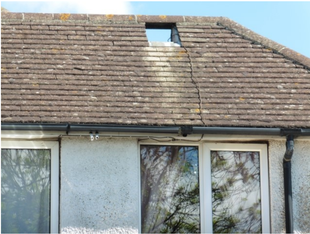
Rear roof pitch
