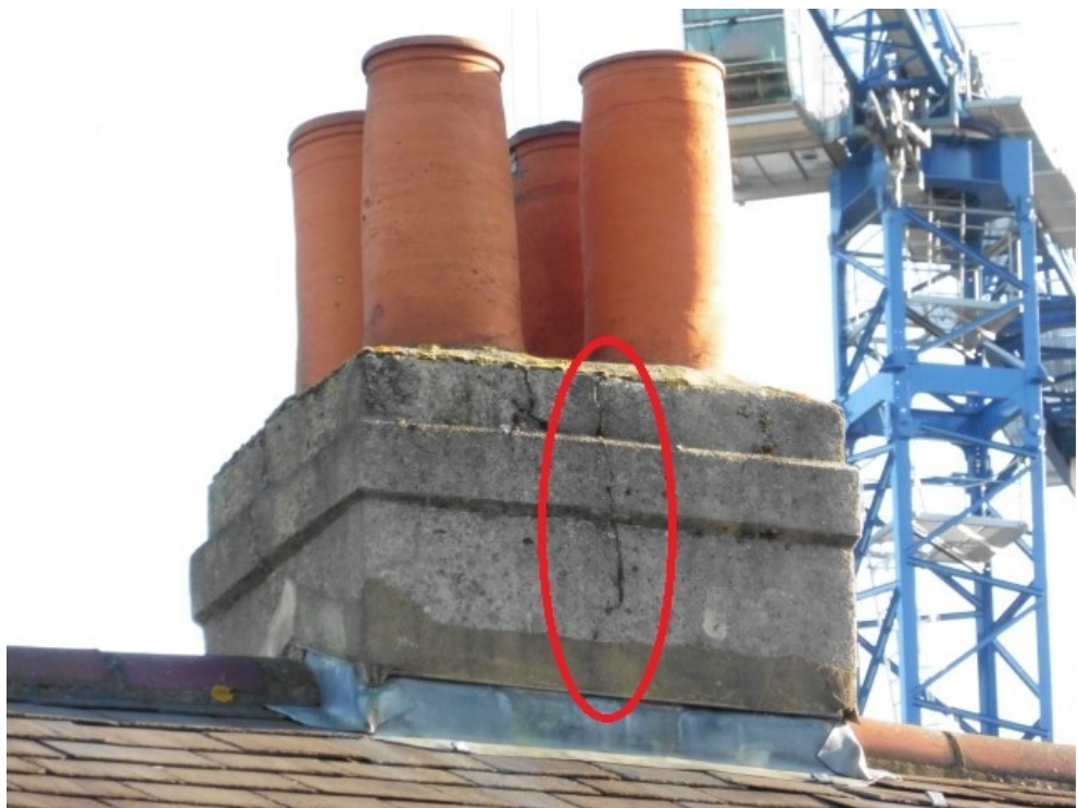
Central stack viewed from the front
