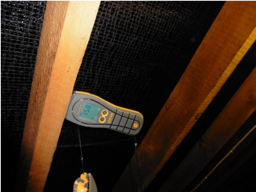
Normal moisture reading in roof timber
